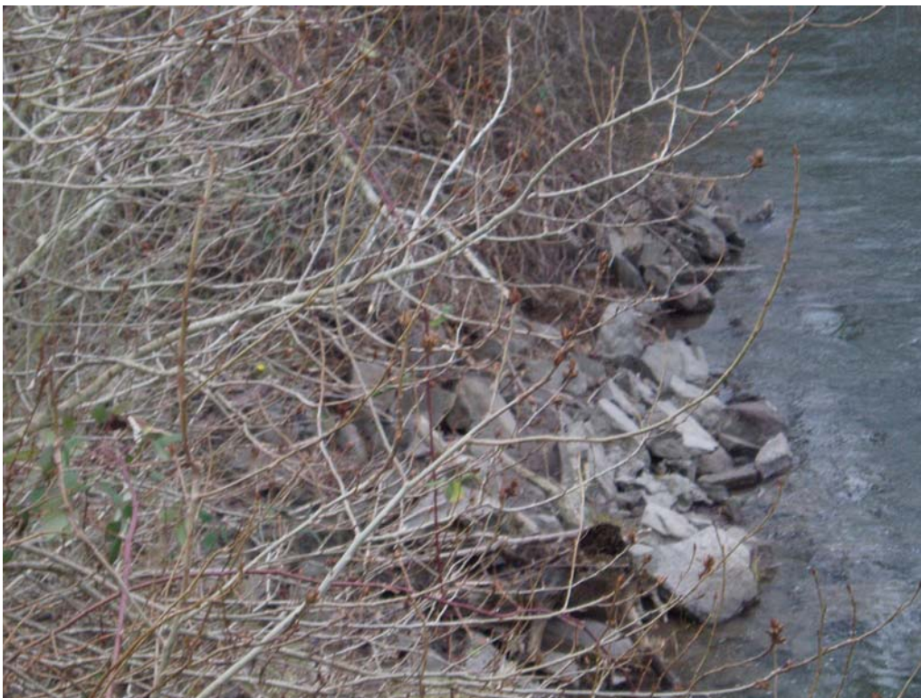
Figure 6.12. Rip rap protecting right bank of west distributary just downstream of the fork of the distributaries.
