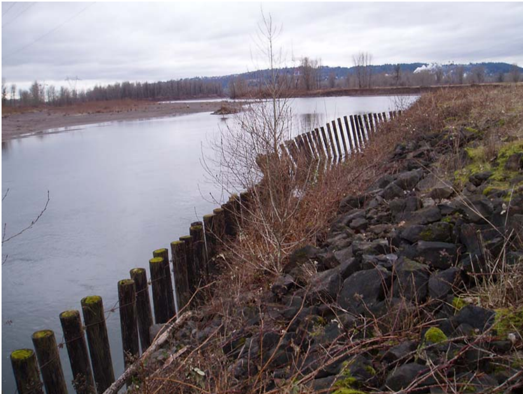
Figure 6.10. Bank protection on right bank of west distributary.
