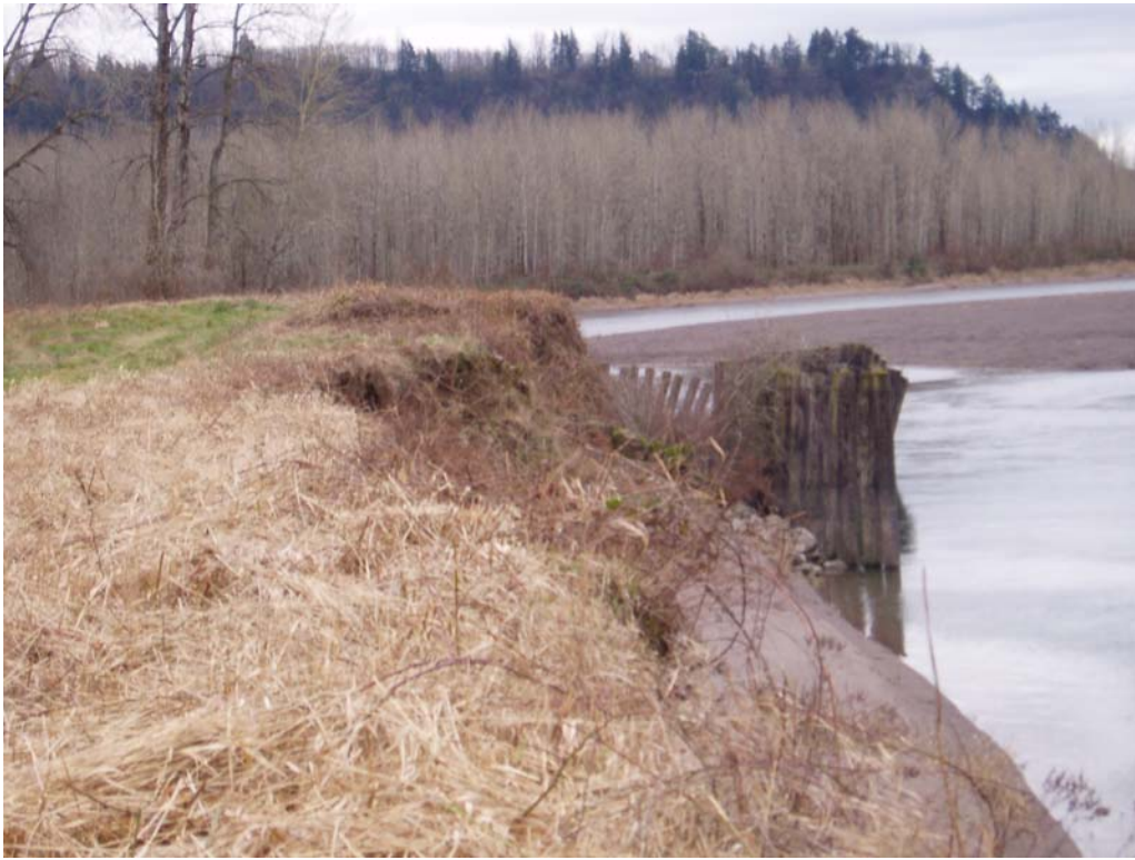
Figure 6.9. Edge of bank protection composed of wooden piles and rip rap.
