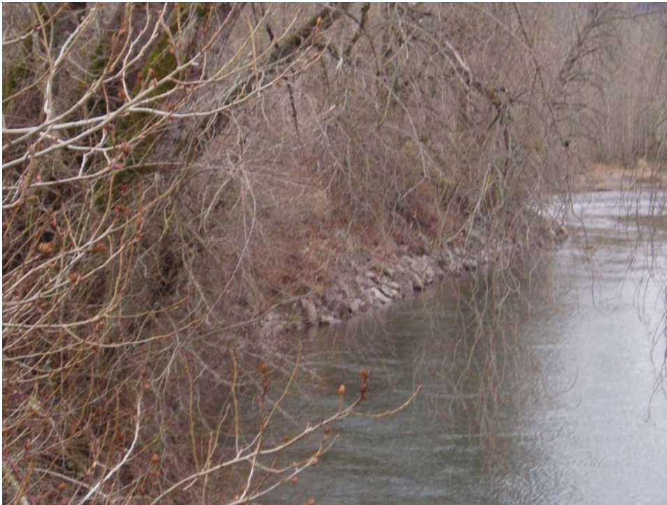
Figure 6.11. Bank protection composed only of rip rap. Note the established vegetation.
